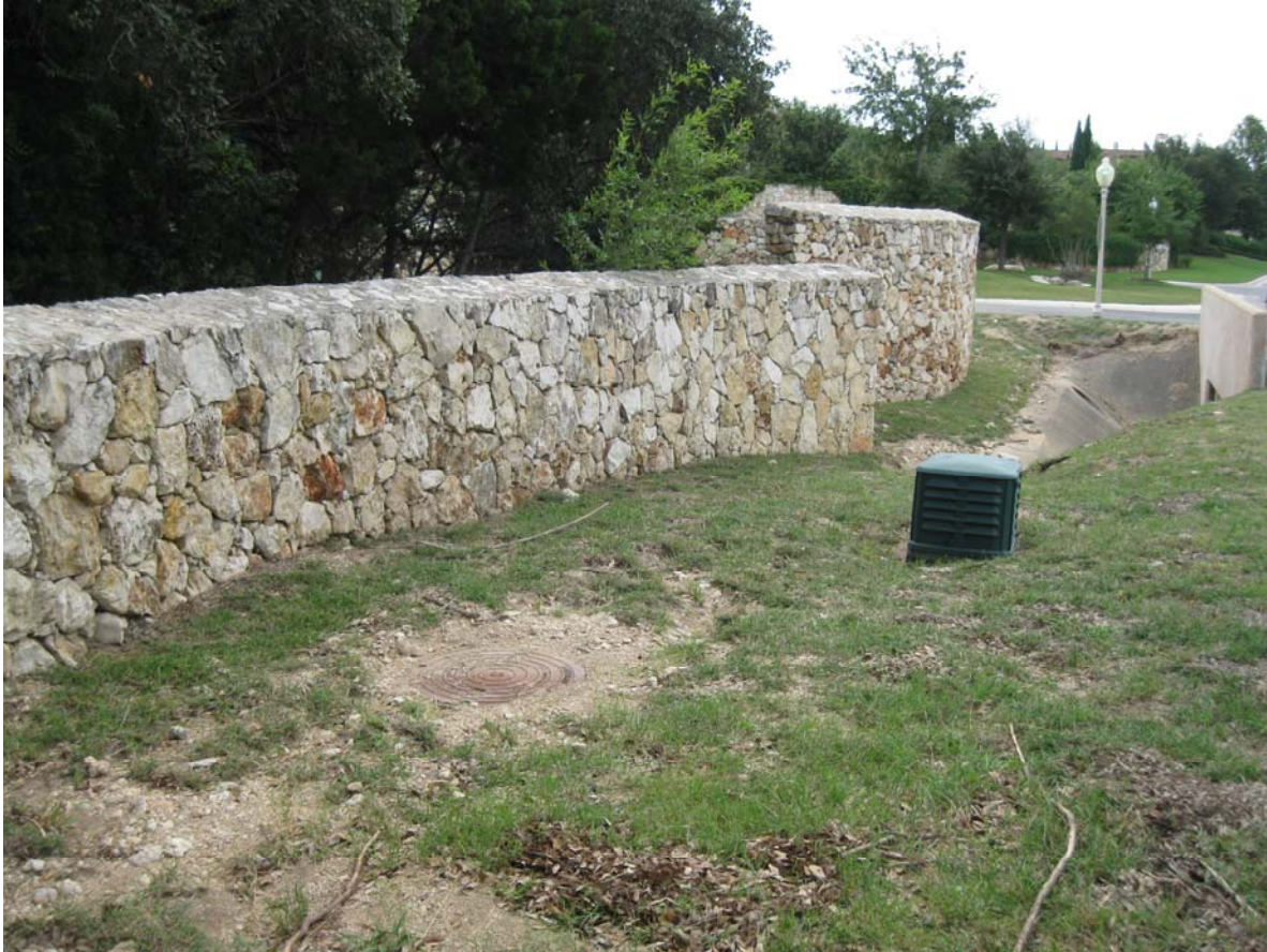
Existing Wall Photo No. 1
