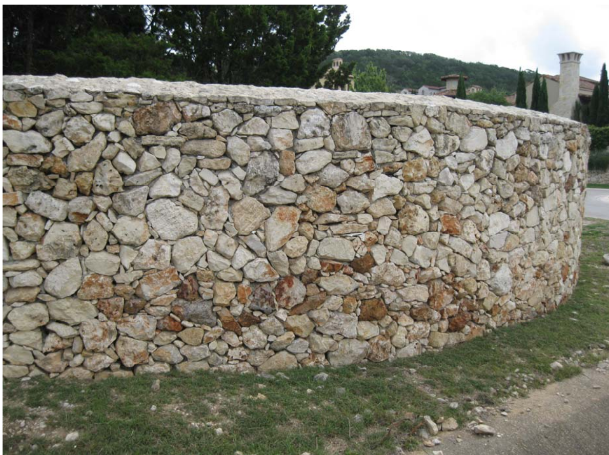
Existing Wall Photo No. 2
